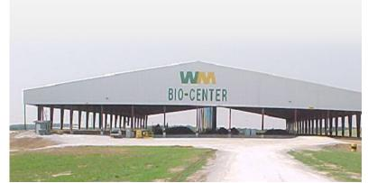
On-site treatment of excavated soil in aerated biopiles
