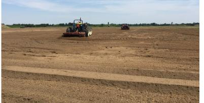
On-site treatment of excavated soil in HDPElined biocell
